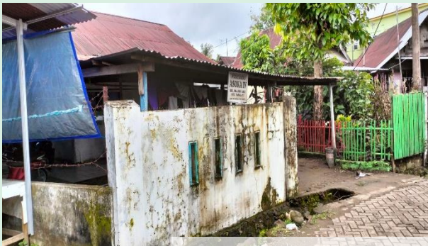
The polyclinic before renovation
